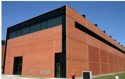
Figure 2. Civil Engineering Department.
